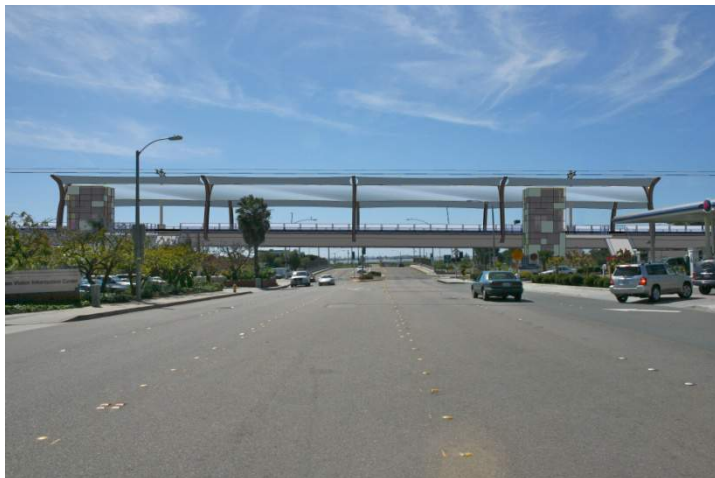
Figure 2: E St. looking west at simulation of station over street.
