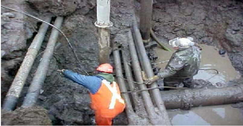
Sewer Rehabilitation - $2.2 million
