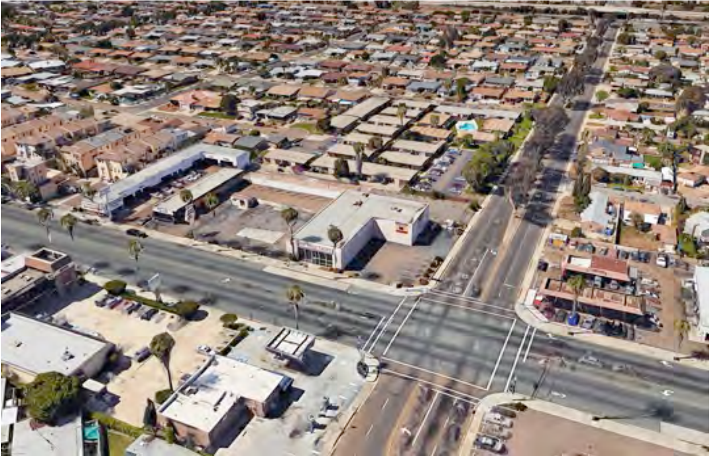
This Google Earth view of the intersection of Broadway and J Street shows the southwest corner lot recently sold by Tom Spencer still occupied with the buildings that would soon be demolished for the construction of the Goodwill store. The large L-shaped building built in 1970 for Carpet Town was leased to Fox Tool Sales, and on the left side of the parking lot next to Courtney Tires is the rectangular building built in 1960 for Tyson Plymouth.
