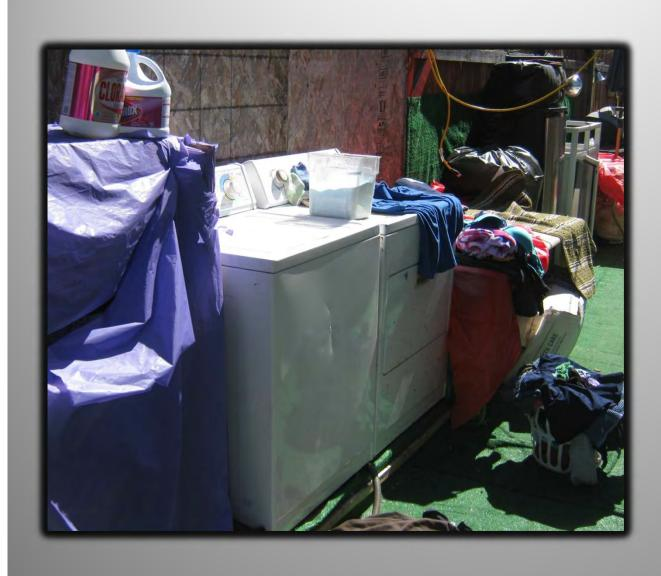
Appliances shall not be installed outside of the unit exposed to the weather or connected with an extension cord. Relocate the appliance(s) out of the weather and/or remove the extension cord. [25 CCR 1134(a), 1188(b), (d)]
