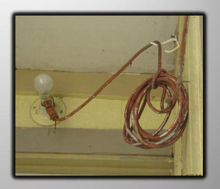
Extension cord is being used to supply power to a source that requires a permanent wiring method. Remove the extension cord and rewire using an approved permanent wiring method. [25 CCR 1188(b),]
