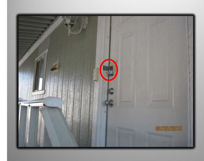
One or more required exterior egress doors are blocked or locked with an exterior hasp, preventing emergency exit. Remove the material or hasp from in front of the doors and provide for proper exiting. [25 1606(c), 1607(c), 1608(c)]
