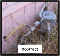
More than one gas supply connection provided to the unit. Remove additional supply line [25 CCR 1354(c)]
