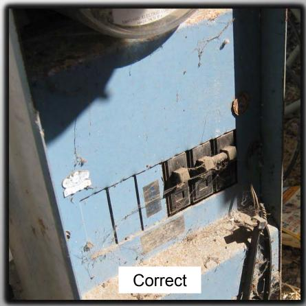
The lot/park electrical service equipment has exposed or easily accessible live electrical parts. Cover all exposed live electrical parts and plug unused openings in electrical equipment. [25 CCR 1134(a), 1188(b); Reference: California Electrical Code, Article. 230-62]
