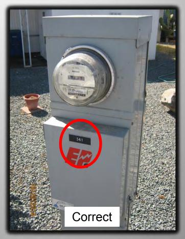
The electrical distribution panels, overcurrent devices, fuses or switches which serve the space, fixture, device or other equipment controlled at the distribution panels are not clearly and permanently marked. Clearly and permanently mark electrical distribution panels, overcurrent device, fuses or switches to identify the space, fixture, device or other equipment controlled at each distribution panel. [25 CCR 1134(a), 1151; Reference: California Electrical Code, Article 110-22, 230-70]
