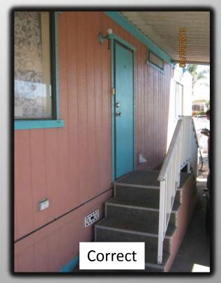
The stairway and/or landing is structurally unsound. Floor of the exterior landing shall not be more than 1 inch lower than the bottom of the outswing door. Replace or reconstruct the stairway and/or landing. [25 CCR 1498(a)(b), 1608(b)]
