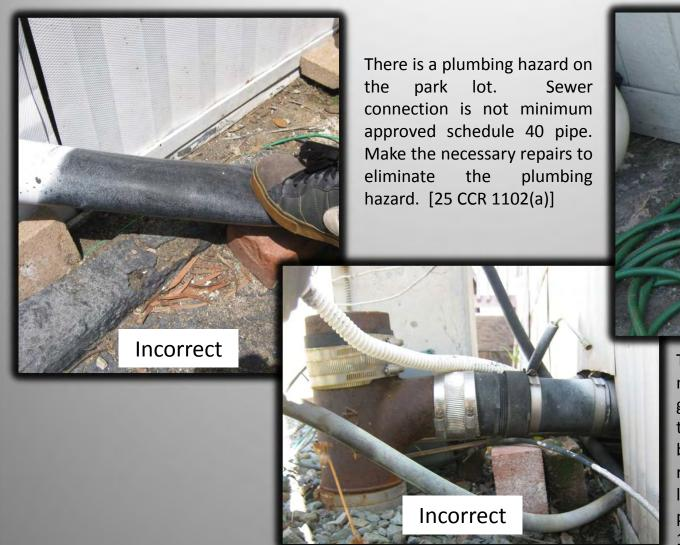
The drain line system is not maintained with a proper grade. A grade of not less than 1/8 inch per foot between the mobilehome or recreational vehicle and the lot drain inlet must be provided. [25 CCR 1358(d), 1606(e), 1607(e)]
