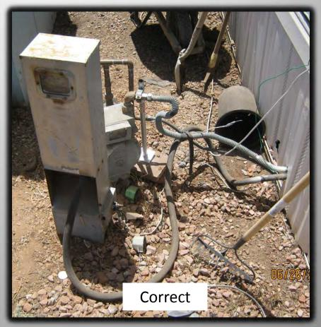
The power supply cord is buried in the ground or encased in concrete. Remove the dirt or concrete covering and if deteriorated, replace the power supply cord. [25 CCR 1188(b), 1352(g), 2352(f)]
