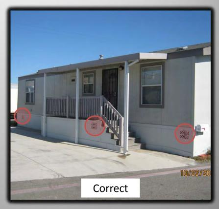
When installed, skirting must have adequate cross ventilation on at least two opposing sides along the greatest length of the unit. [25 CCR 1346]
