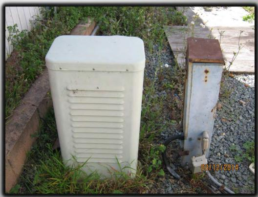
The park/lot electrical service equipment is not accessible for inspection, repair, or disconnection in case of emergency. Provide unobstructed working clearance of at least 30 inches wide by 30 inches deep and 78 high in front of the electrical equipment. [25 CCR 1183; Reference: California Electrical Code, Article 110-26]
