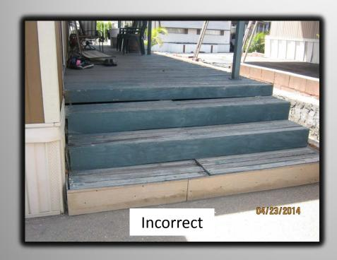
The porch and/or deck is constructed 30 inches or more above the ground and does not have a guard rail. Provide a guardrail around the perimeter of the porch and/or deck, no less than 42 inches above the floor of the porch and/or deck. [25 CCR 1502; Reference: California Residential Code R312]
