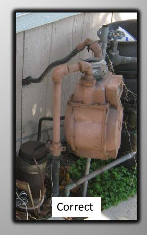
The gas meter provided on the lot has been enclosed or obstructed in such a manner as to restrict ventilation to the gas meter. Remove enclosure or obstruction to provide accessibility and ventilation to the gas meter. [25 CCR 1226(b)]
