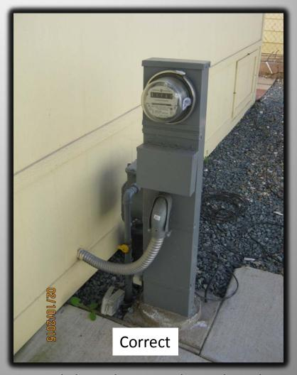
The MH-unit electrical supply conduit is buried or in direct contact with the earth. Uncover the supply conduit and support above grade. [25 CCR 1352(e), 2352(f)]
