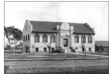
Chula Vista's Carnegie Library, built in 1917 and demolished in 1960. Image Source: City of Chula Vista Public Library and Heritage Museum.
