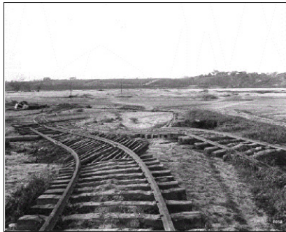
Coronado Railroad Lines at Chula Vista damaged from the 1916 flood. Image Source: City of Chula Vista Public Library and Heritage Museum.
