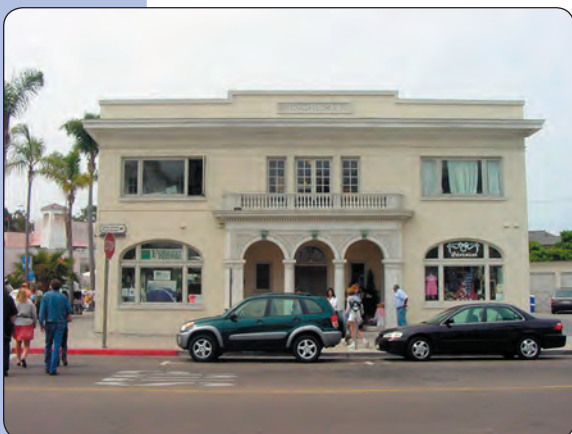
Arches should be semi-circular and relate to the scale of the building
