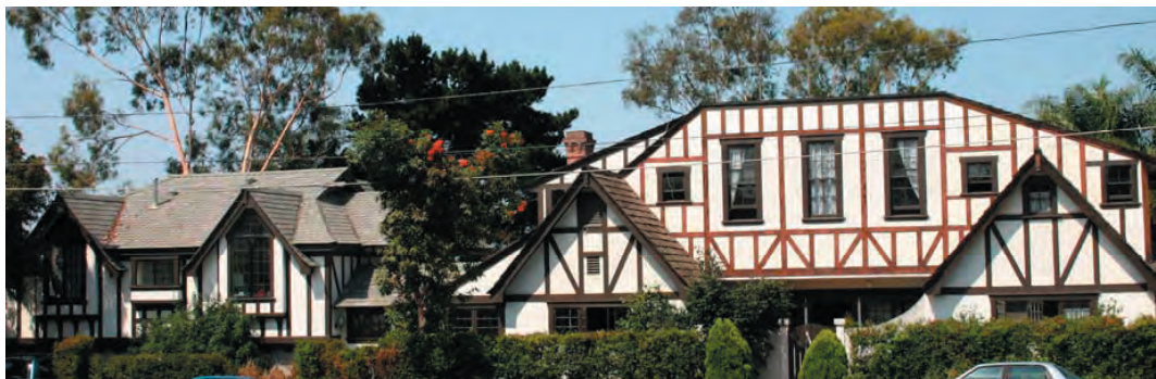
Mae Edgecomb House Tudor Revival, ca 1924 834 First Ave
