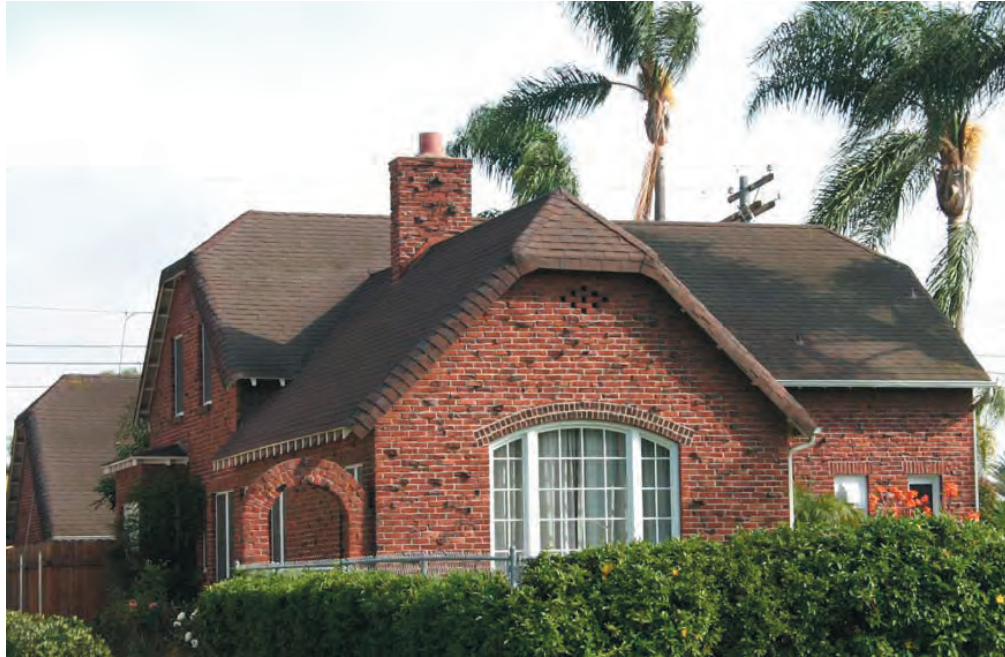
Horace Nelson House, Historic Site # Tudor Revival brick house, 1933 470 "E" St
