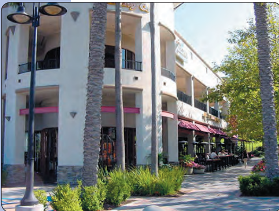
Masonry is appropriate for buildings in the Urban Core Fig. 7.110
