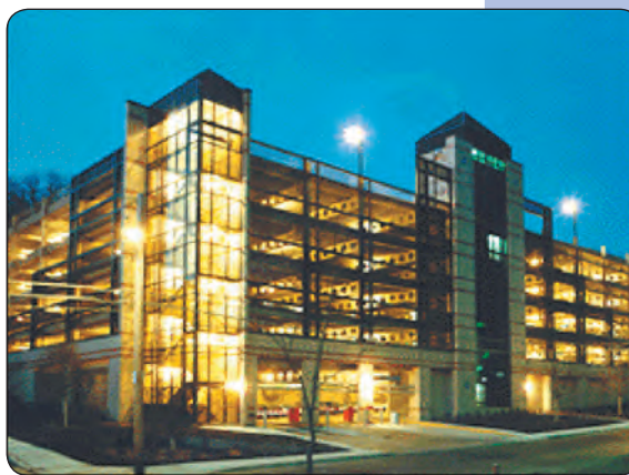
Open lobbies and stairs promote safety in parking structures
