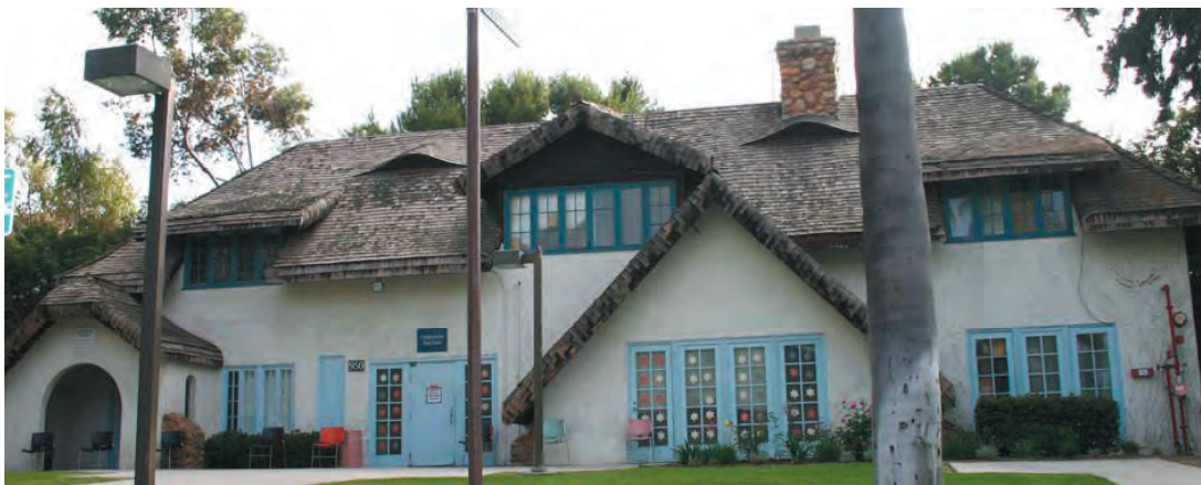
Bay View Hospital Tudor Revival, Third Ave at "L" (half-timbers were stuccoed over)
