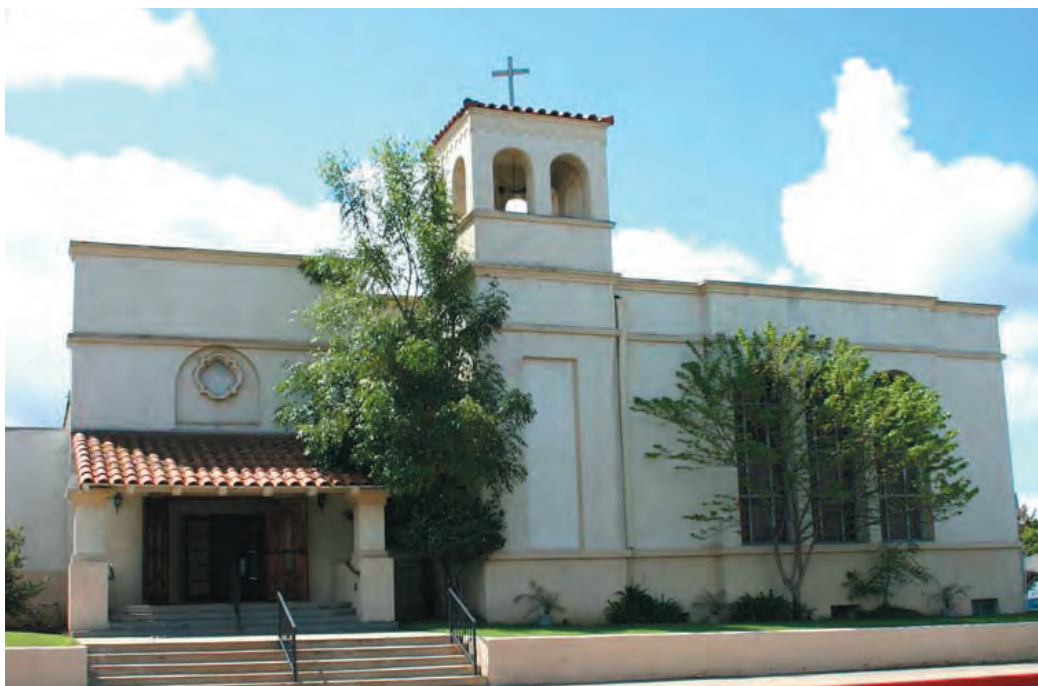
First Baptist Church of Chula Vista, 1929 Spanish Colonial Style "E" St & Fifth Ave
