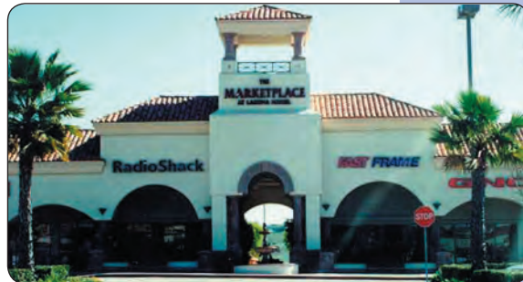
Vertical elements such as a tower are encouraged
