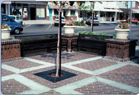
Tree grates are important in high-traffic areas
