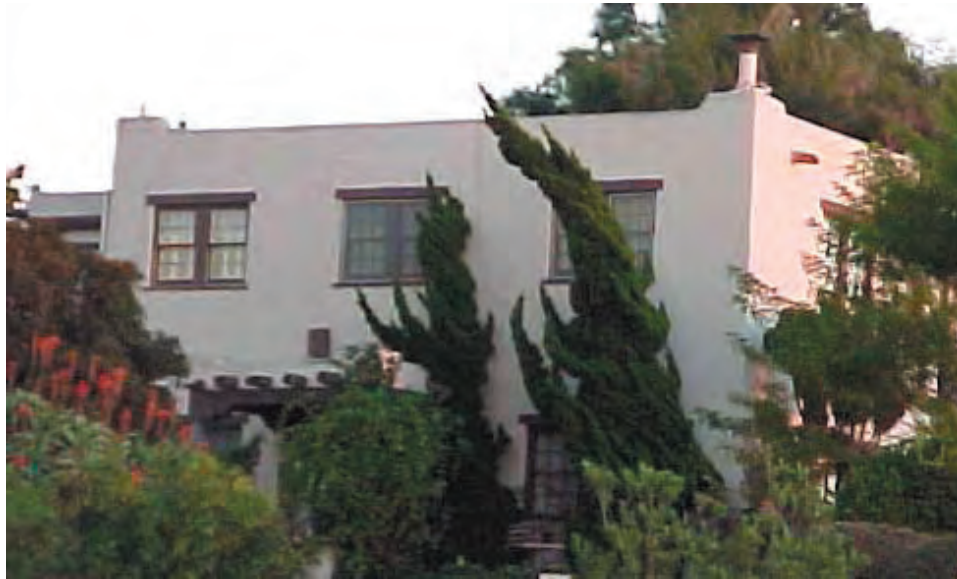
Sallmon House, 1916, Pueblo Revival Style Designed by William Templeton Johnson in 1916 Historic Site #28 435 First Avenue
