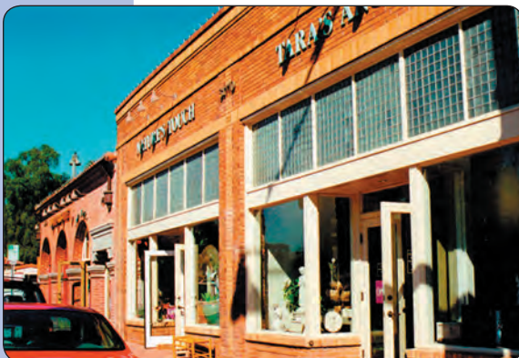
Transom windows increase the amount of natural light inside Fig. 7.69
