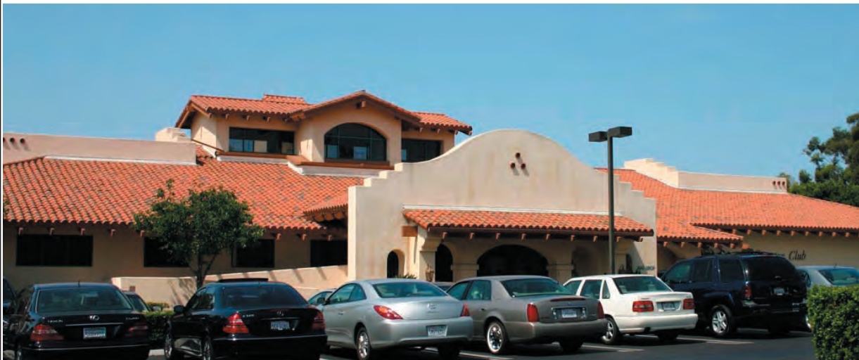
San Diego Country Club, 1984 Pueblo Revival Style "L" Street Chula Vista
