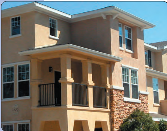
Upper floor balconies and windows overlooking the street are provided Fig. 7.194
