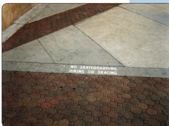
Special accent paving can be used on sidewalks
