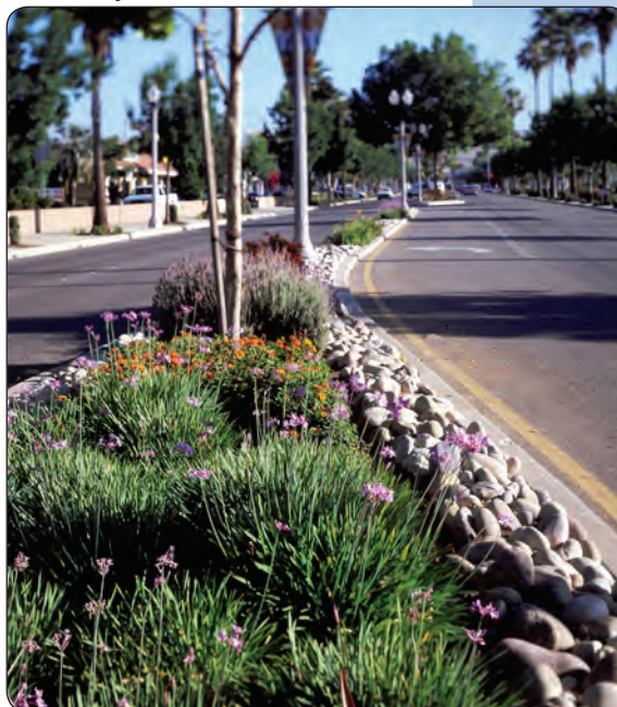
Medians should provide a maintenance strip as a buffer
