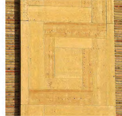
Concrete Paving with Roman Brick Banding
