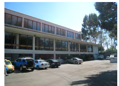
Library Administration, central services, and building support areas are located on the lower level of the Civic Center Branch.
