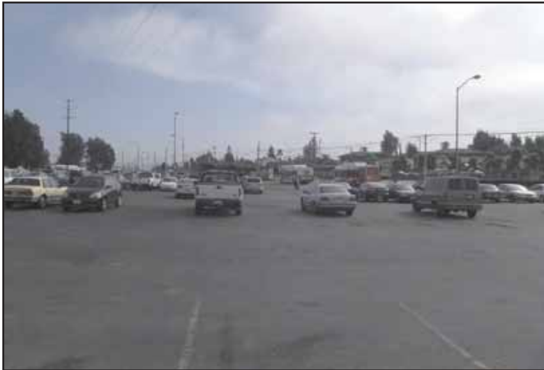
Photo 3 – Palomar Transit Station parking lot
