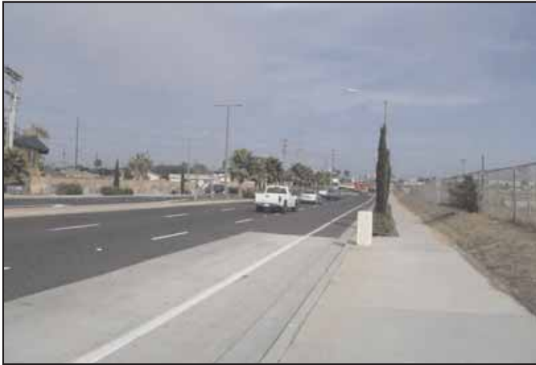
Photo 1 - View looking east along Palomar Street from Frontage Road
