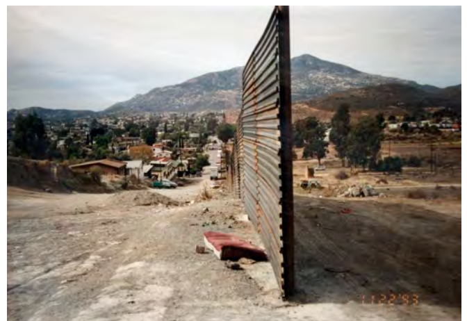
Surplus military landing mat being installed in 1993.
