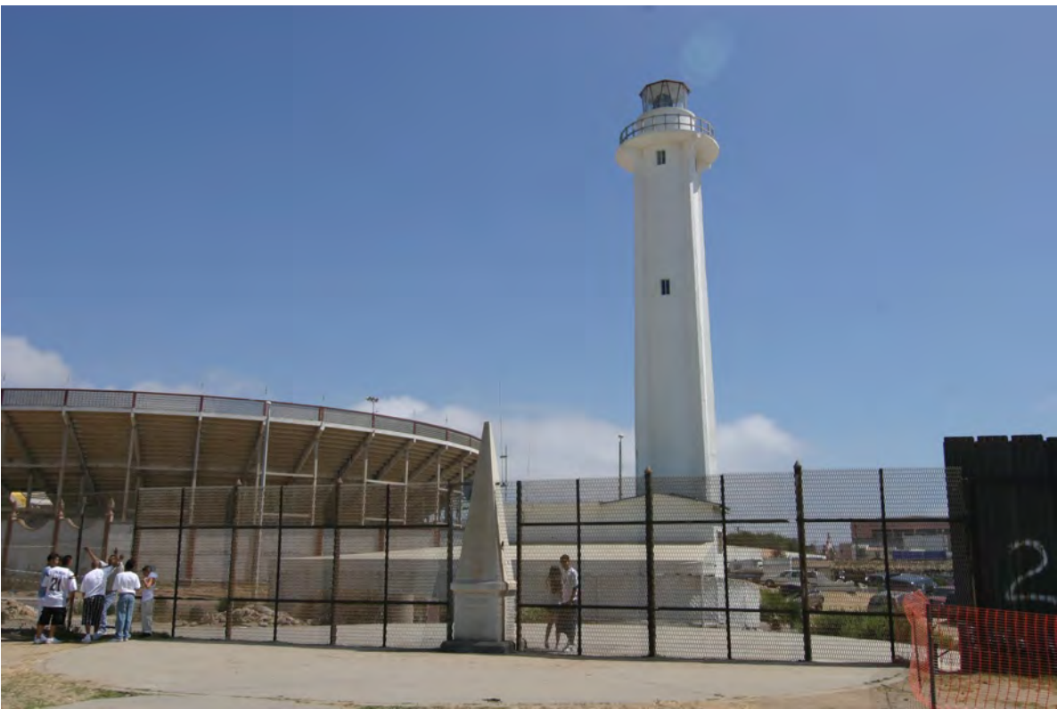
Above, Monument No. 258 in 2008, and below in 1976 showing the old barbed wire fence from the 1940s that was replaced by the tall metal fence in 1994.
