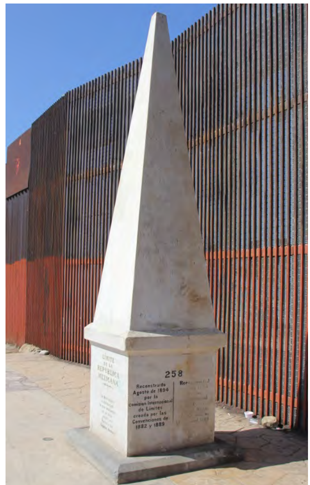
Monument 258 in 2015, viewed from the Mexican side, with military surplus landing mat fence installed in 1996.
