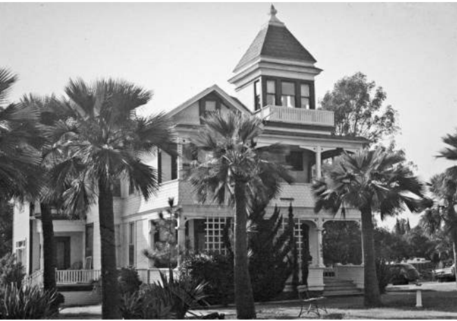
example of Queen Anne architecture with its prominent finial spire and widow's walk. The house features the high hip and steep gable roof often found on homes of this style. The roof has a boxed cornice and a plain frieze. Other details include an exterior
