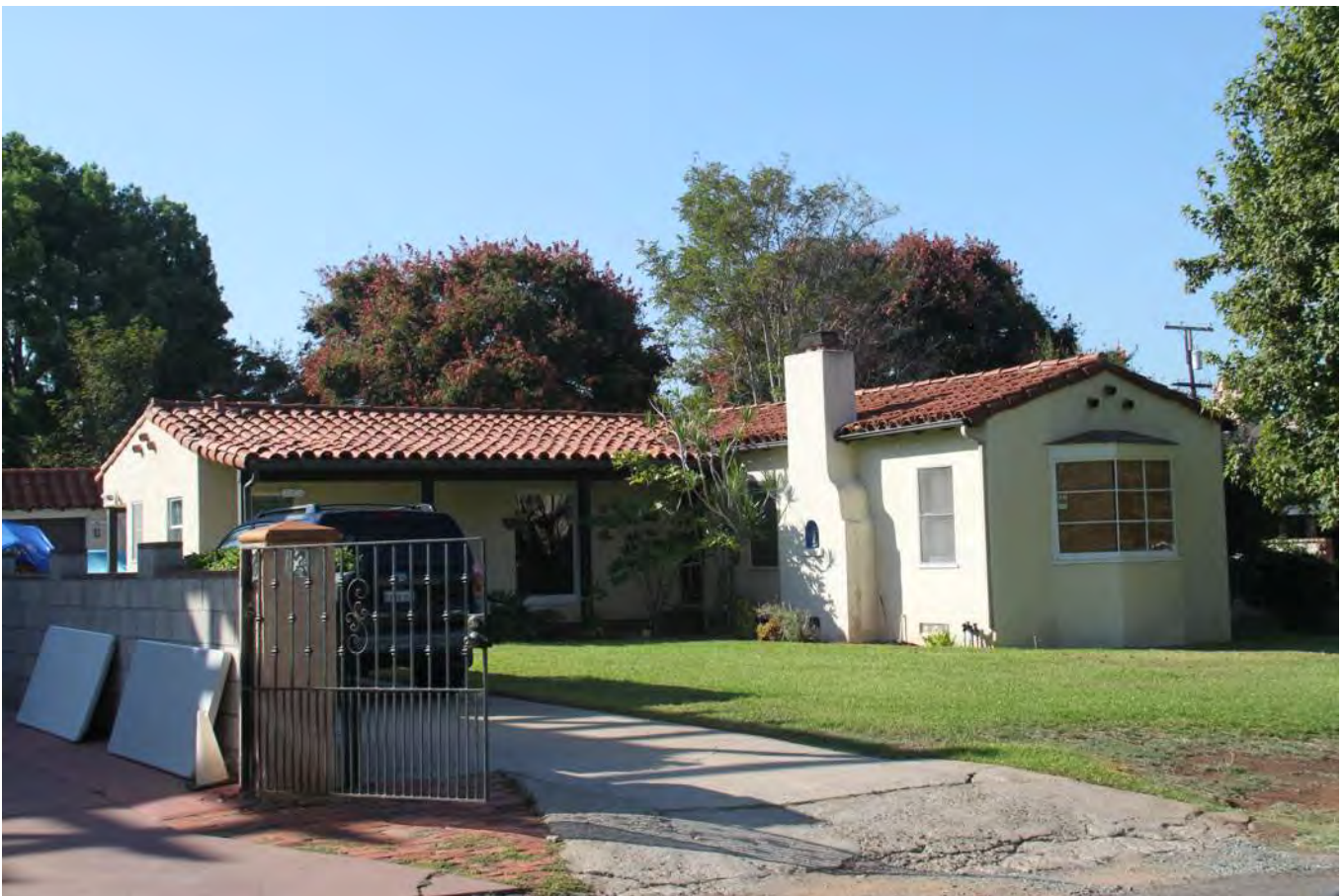
The Markey House at 206 Bayview Way in the Clare Haven subdivision has recently been designated as Chula Vista Historic Site No. 101.
