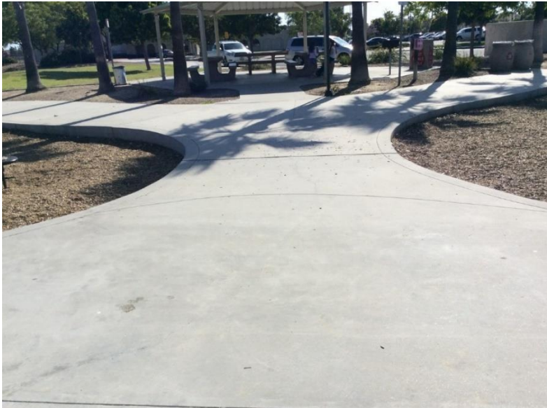
Figure 2-14 Pedestrian Walkway - Condition 2
