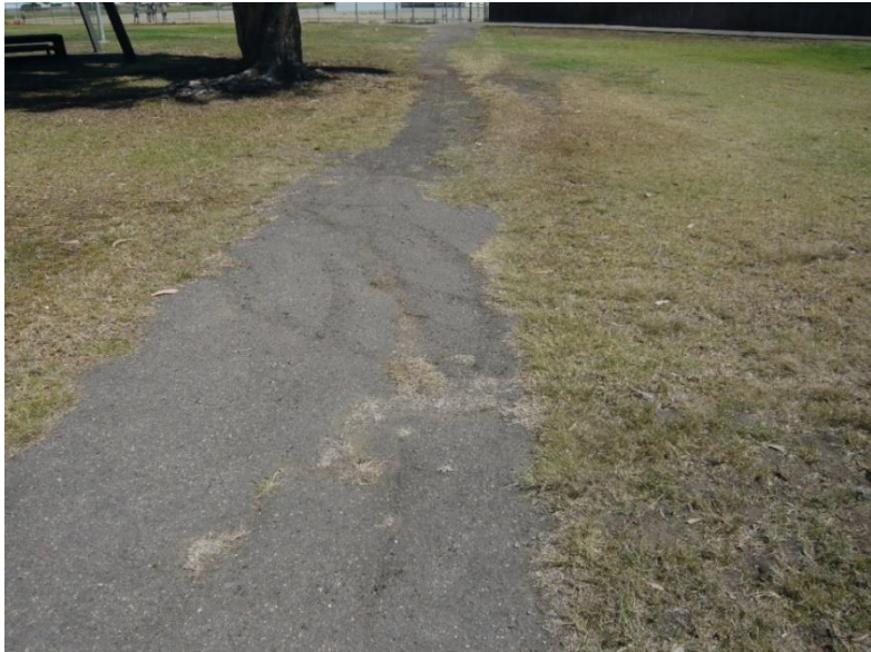
Figure 2-13 Pedestrian Walkway - Condition 5
