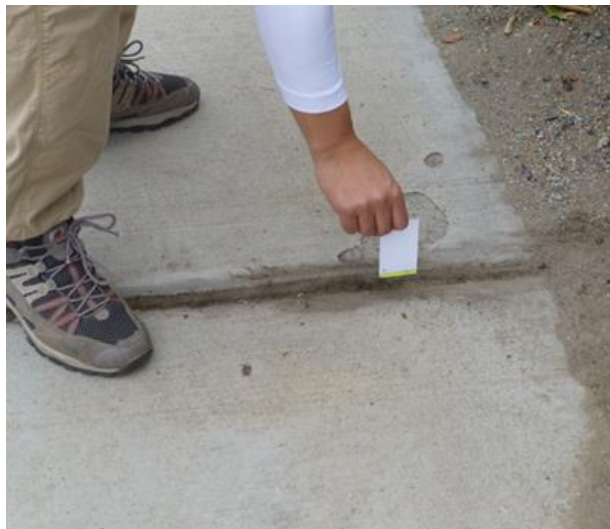
Figure 2-9 Sidewalk Condition Assessment
