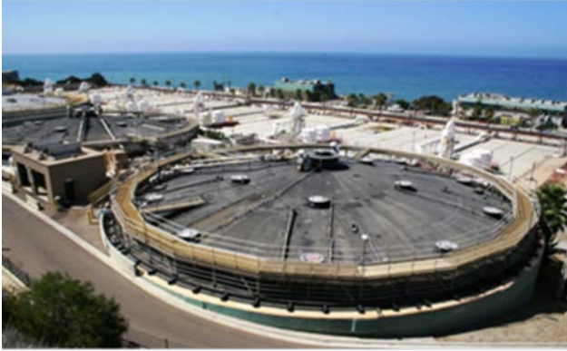
Pictured above: Point Loma Treatment Facility
