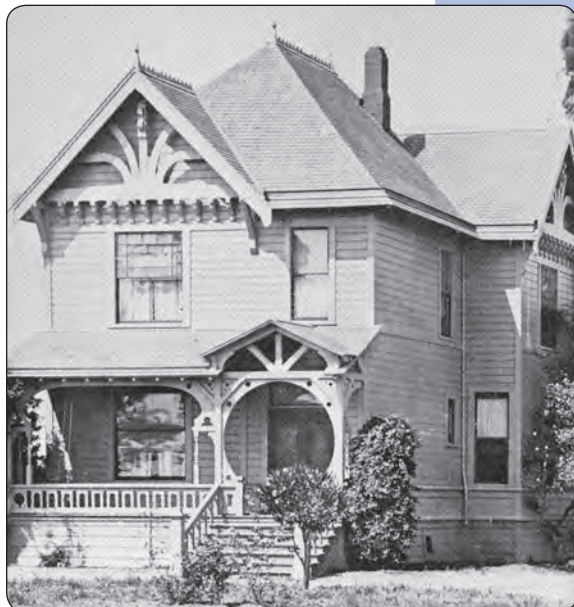
Photo of “Our House” before it was destroyed by fire
