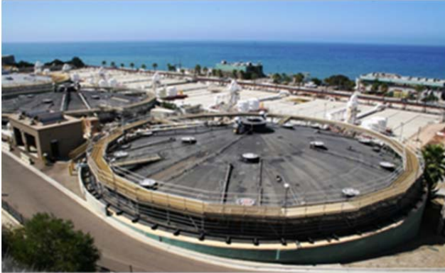
Pictured above: Point Loma Treatment Facility
