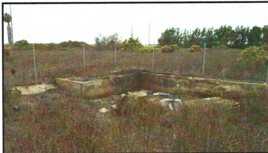
Photograph 1: View of concrete lined basin, looking to the northwest.
