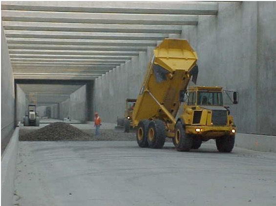
Stage 3: Ballast placement
