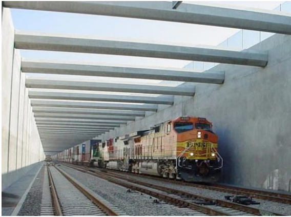
Stage 4: Completed trench
