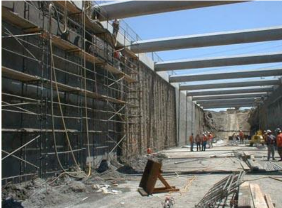
Stage 2: Construction of invert slab and wall facing
