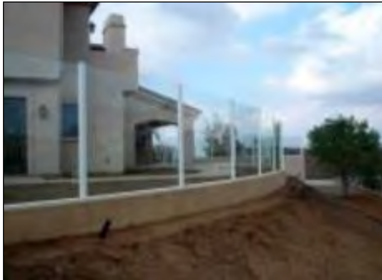
Figure 22. Example of Heat Deflecting View Wall
