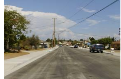
Glenhaven Way Improvements
