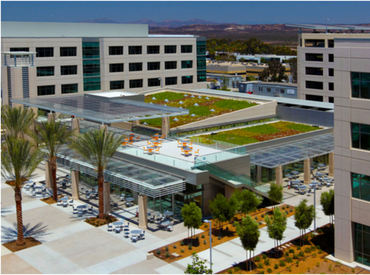
Location: County of San Diego Operations Center, San Diego, Ca
