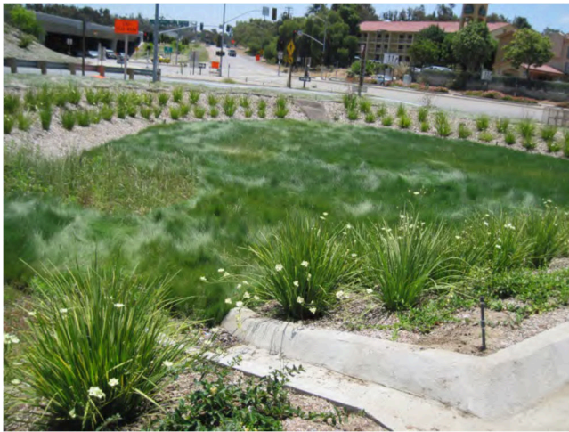
Location: 805 and Bonita Road, Chula vista, C.A.
