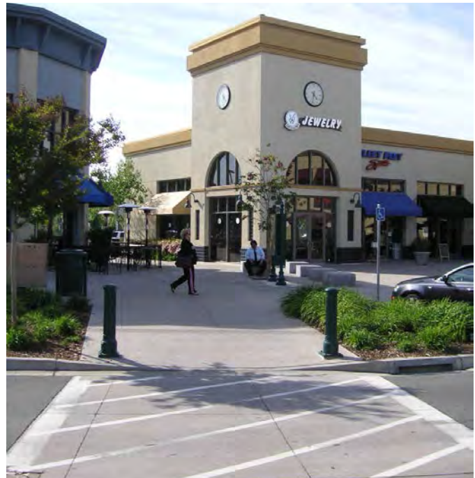
Pedestrian crossing with landscape bulb-out, bollards, and striping to promote safe pedestrian crossings.
