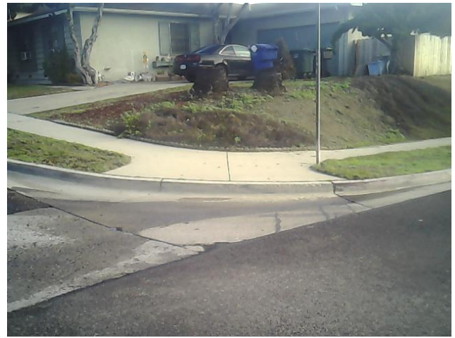
Missing Curb Ramp
