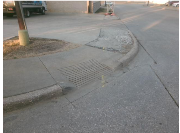
Curb Ramp Running Slope
