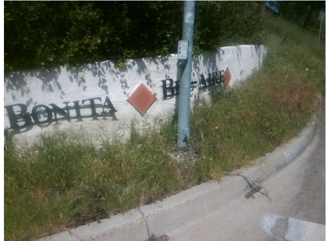
Pushbutton Clear Floor Space - Missing
