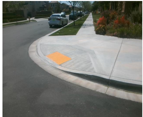
Curb Ramp with Detectable Warning Surface
