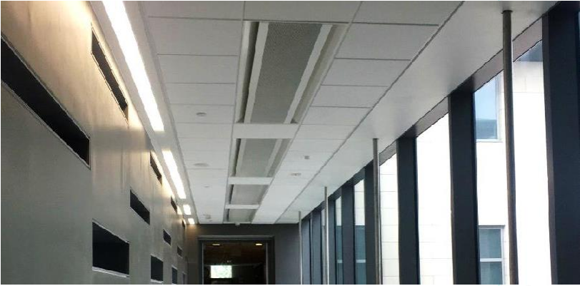
↑ Chilled Beams
