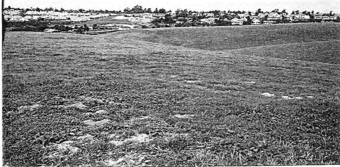
Northern Portion of Site, looking Northeast Toward Eastlake
