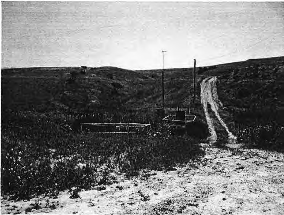
Photograph #5 Aqueduct tunnel structures at base of Wolf Canyon looking south.
