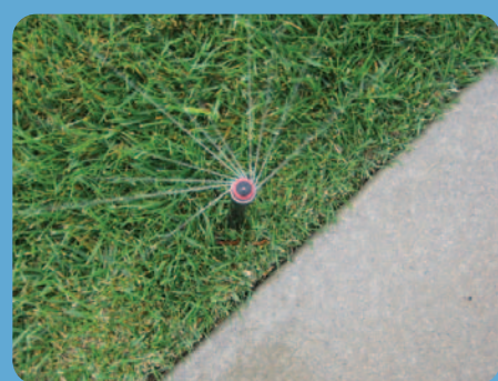
A rotating nozzle is easy to install in existing irrigation systems and reduces the amount of water used by about 20-50%.
