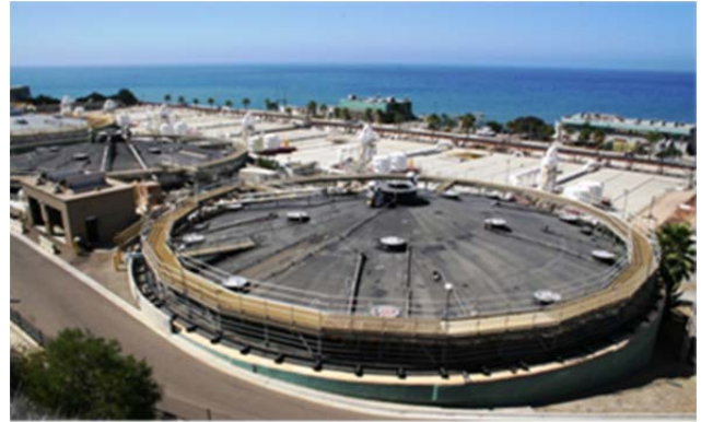
Pictured above: Point Loma Treatment Facility
