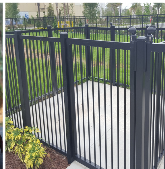
Improved Entry Area
