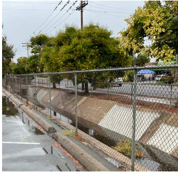
Concrete Stormwater Channel
