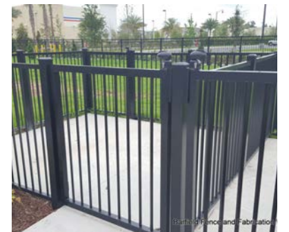
(2) Fencing & Entry Gates
