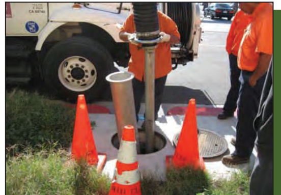
Insertion of vacuum hose into separation chamber.
