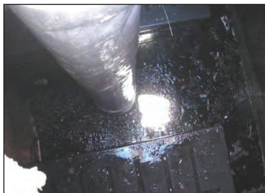
Removal of trash, sediment and debris.
