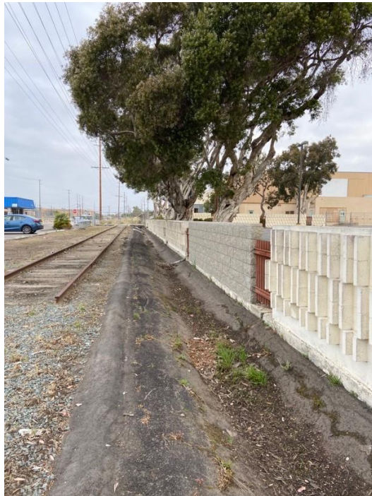
Photo 6. View of asphalt drainage that occurs west of project Planning Area A and east of Planning Area B-1 and Planning Area B-2, facing north.
