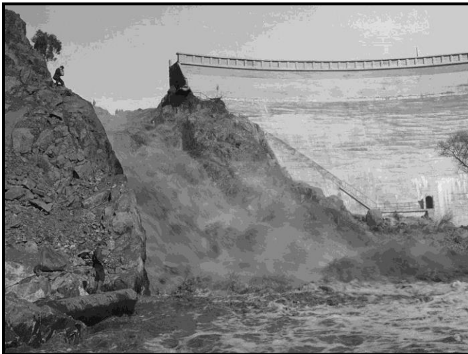
Plate 5: Sweetwater Dam breach in January 1916. (Photograph courtesy of the South Bay Historical Society)
