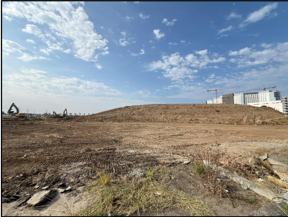
Plate 13: Overview of the project, showing a soil stockpile, facing southwest.
