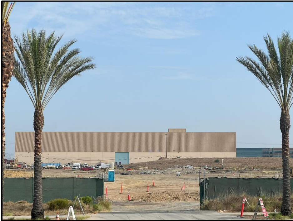
Plate 12: Overview of the project, showing the active construction site, facing north.
