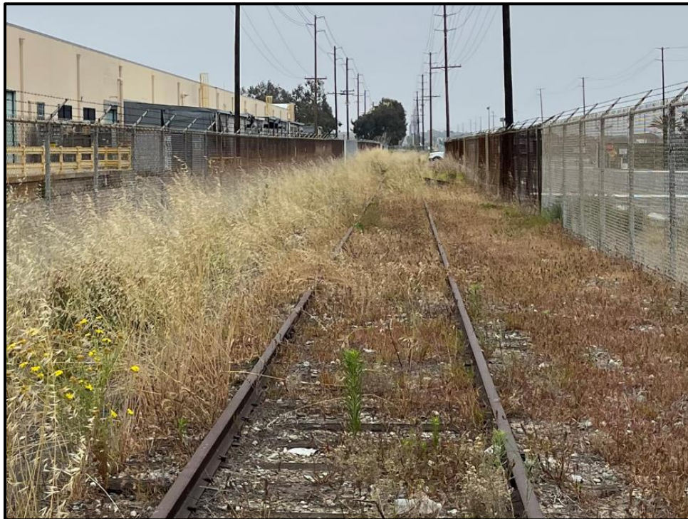
Plate 16: View of Segment D of Site SDI-13,073H between G and H streets, showing the switch at the right of the frame, facing southeast.
