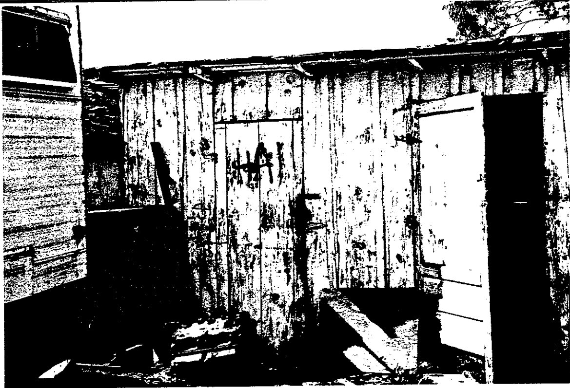
TOOL SHED OF THE SAME PERIOD AS THE BUNGALOW, WAS ONCE THE OUTDOOR LATRINE.
