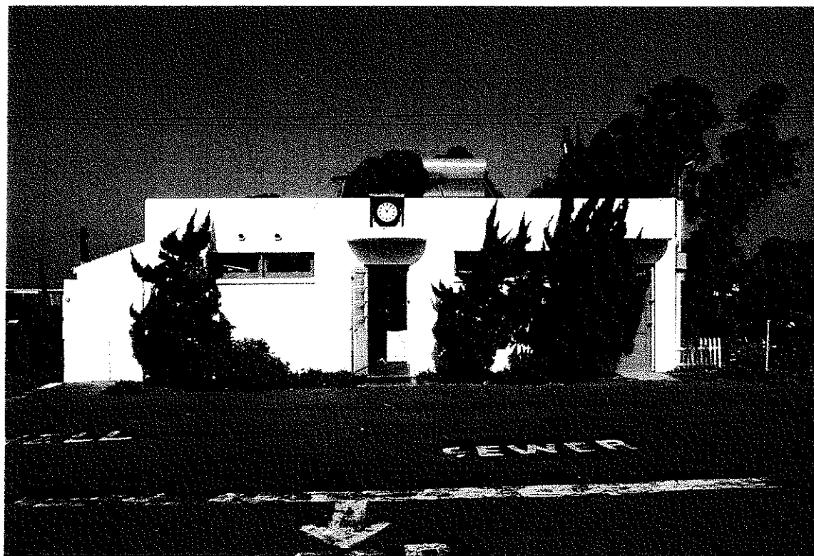
View of the Art Moderne laundry building.
