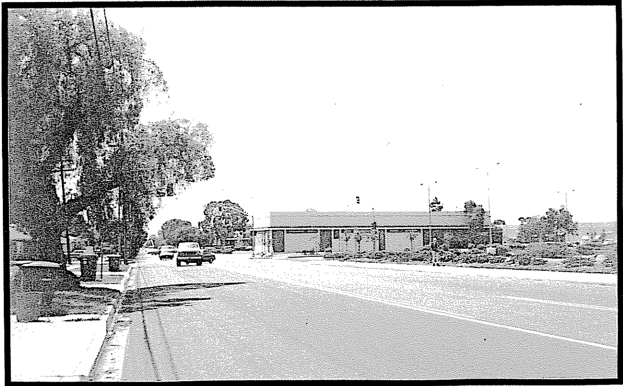
PHOTOGRAPH 5. VACANT J.C. PENNEY AUTOMOTIVE CENTER FROM "I" STREET
