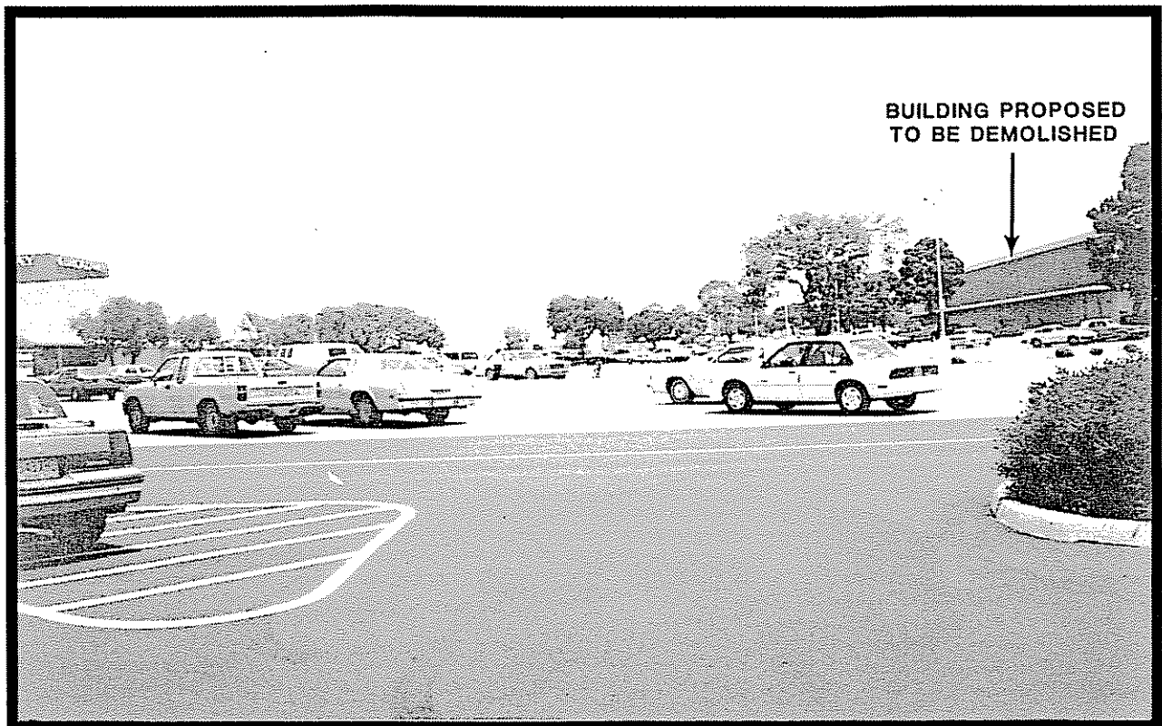
PHOTOGRAPH 9. VIEW LOOKING EAST ACROSS SOUTH SIDE OF MALL
