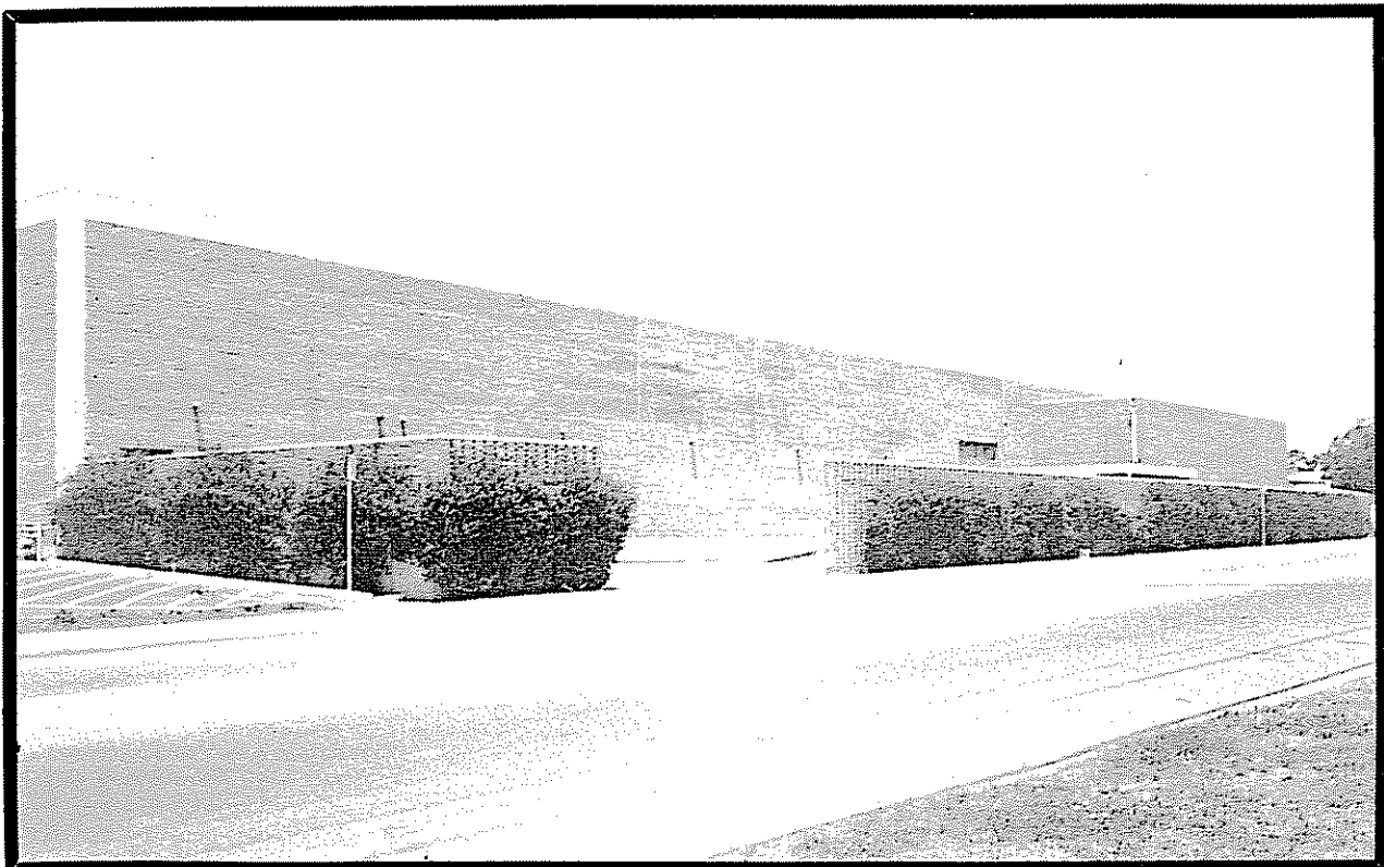
PHOTOGRAPH 4 . REAR WALL OF BUILDING PROPOSED TO BE DEMOLISHED
