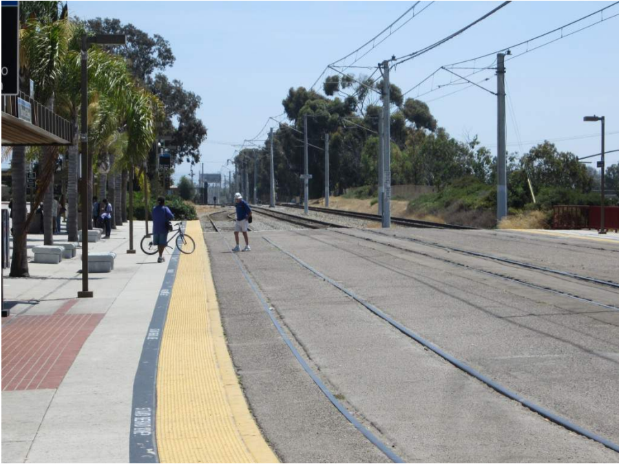
E Street Looking South
