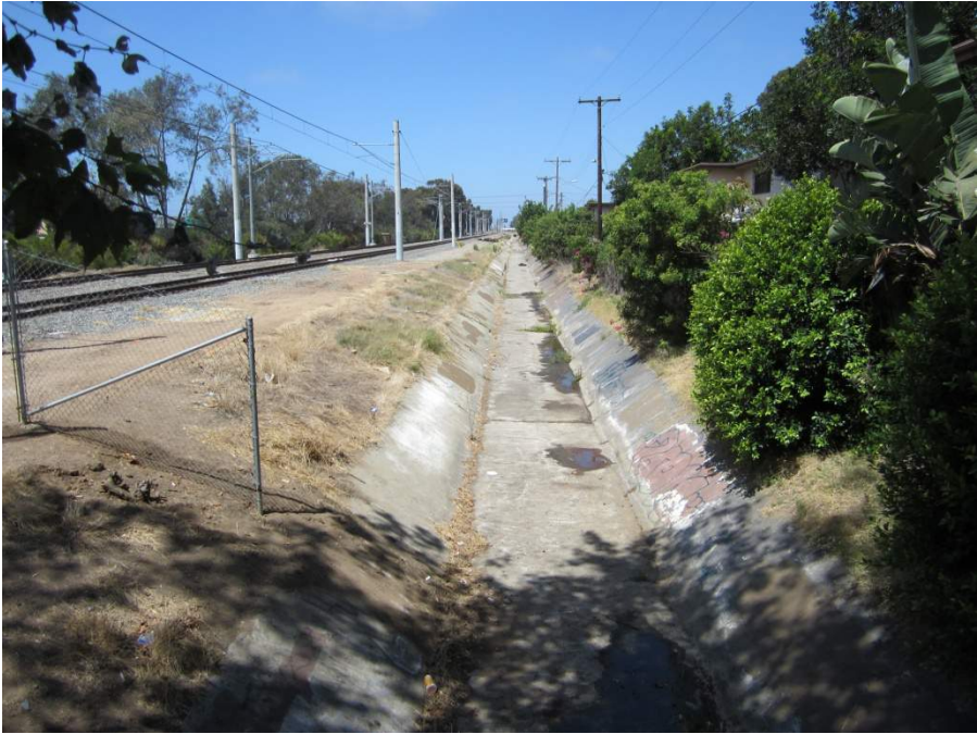
H Street Concrete Lined Ditch Looking North
