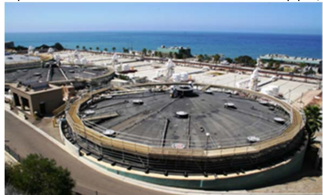
Pictured above: Point Loma Treatment Facility
